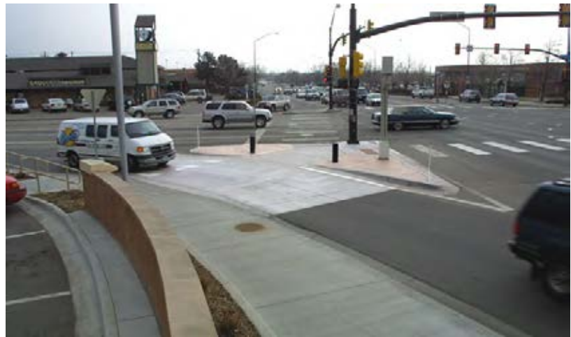
Figure 23 – Example of a ‘pork chop’ refuge island. Note the yield sign and the protective bollards. Source: Dan Burden, CMAP Complete Streets Toolkit
