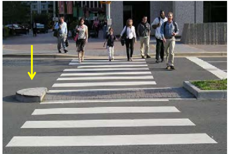
Figure 21- Example of a crosswalk through a median refuge island. Note the nose that extends beyond the crosswalk. Source: NACTO Urban Street Design Guide, 2013.
