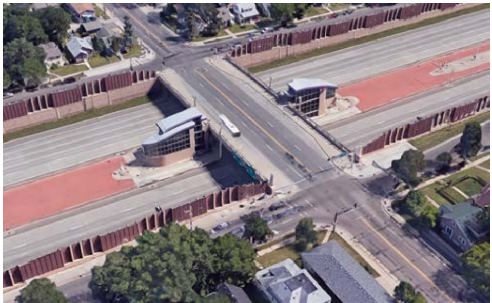
Figure 44 - An example from Minneapolis of a transfer station connecting express buses and local buses. This station is located where I-35W crosses E 46th St. Source: Google Maps
