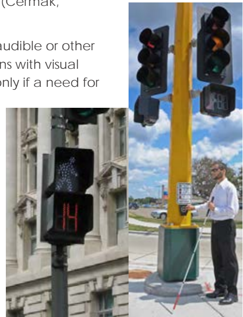
Figure 18 - Countdown Signals and Accessible Pedestrian Signals. Source: IDOT Bicycle and Pedestrian Toolbox and MNDOT
