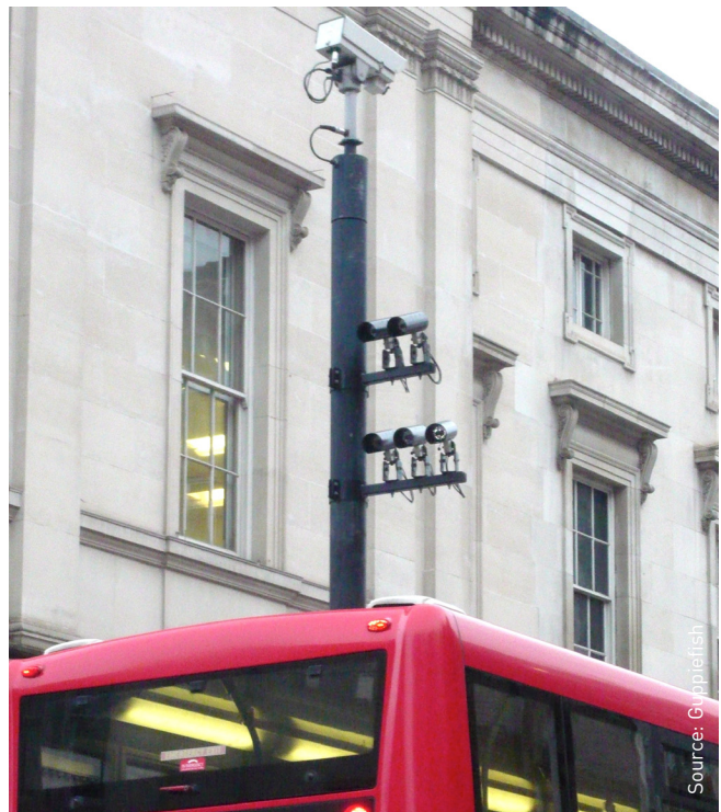
Charging area camera in London
