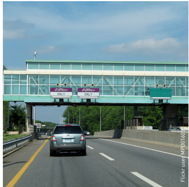
Example of AVI antennas to read transponders and cameras to capture license plates
